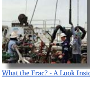
What the Frac? - A Look Inside a Frack Job
